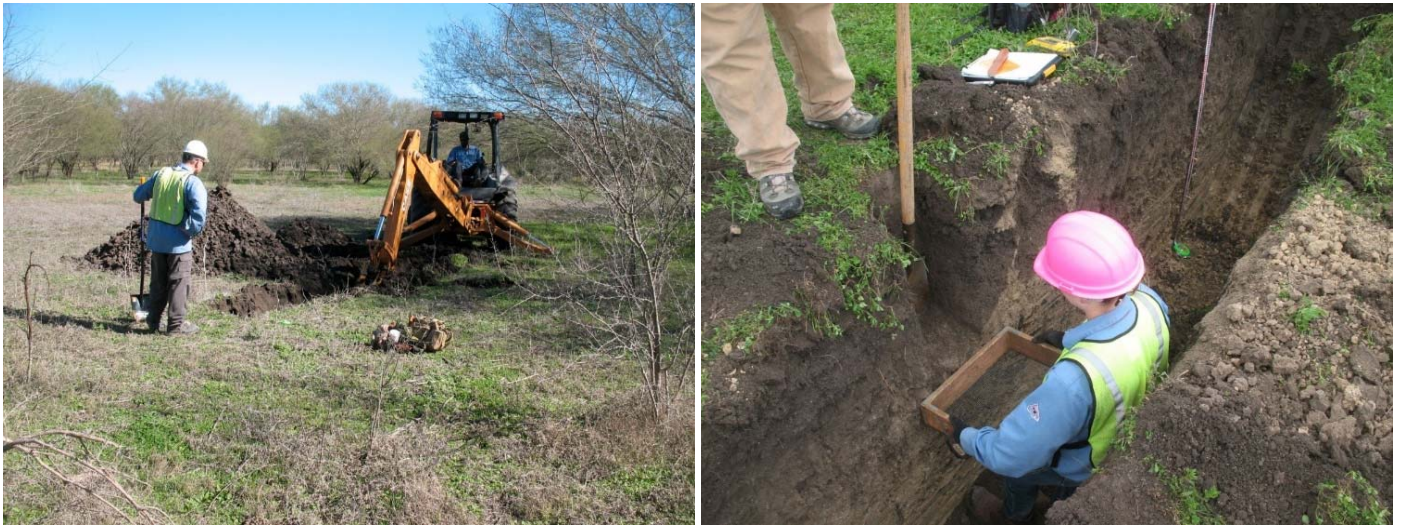
Figure 1. Monitoring trench excavation (left) and excavating a column sample (right).
