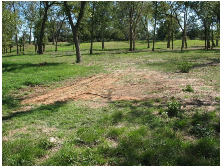
Figure 2. Backhoe trench after completion.
